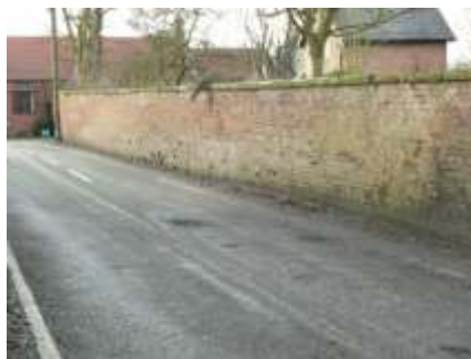
Damage to Wall from road salt Pitted road surface on Church Lane
