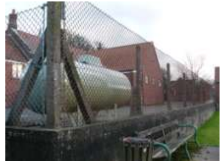
Mesh fencing at Village Hall
