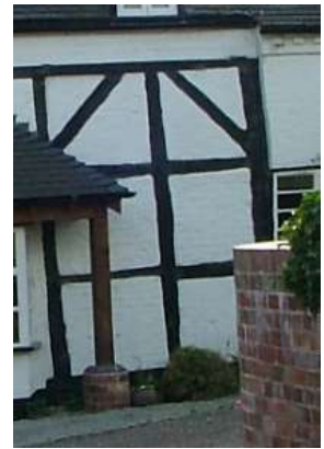
Timber Framing with Brick Infill Panels
