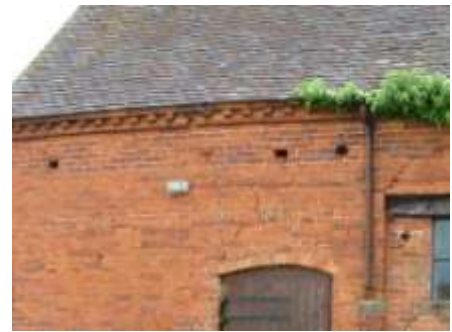
Dentilled gable to barn at Wells Farm Dentilled cornice, clay plain tiles and segmental brick door head at Church Farm
