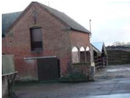
Dentilled gable to barn at Wells Farm Dentilled cornice, clay plain tiles and segmental brick door head at Church Farm
