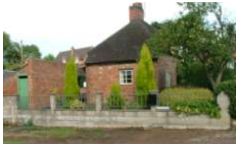
Concrete wall and steel fence to Spring Farmhouse
