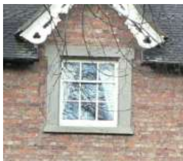
Three-over-six sash window at the Old Vicarage
