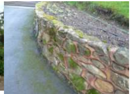
Modern stone wall in front of The Orchard
